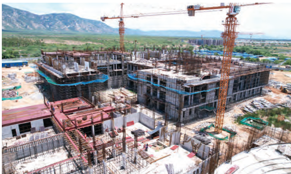
◀ Research block under construction
