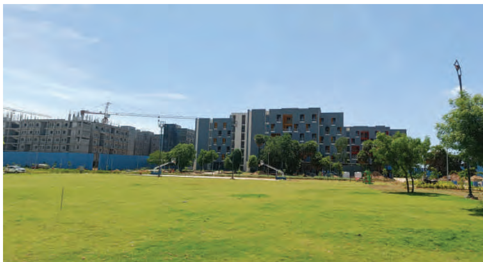
◀ Occupied hostel blocks
