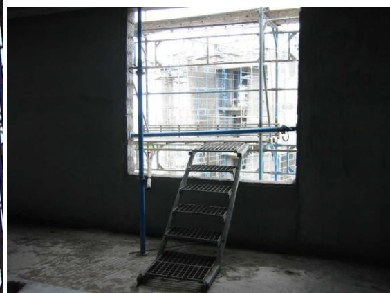
Proper Access to workplatform
